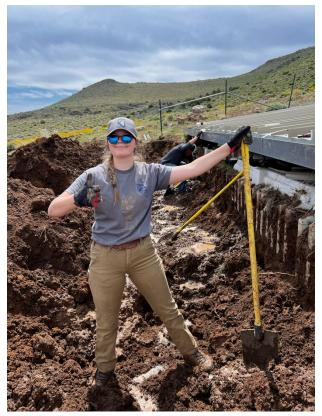
tank system. Guzzler tank systems are all built to utilize the forces of gravity in order to bring water from the storage tanks to the drinker (where animals can utilize this water source). By using gravity, it eliminates the need for a mechanical pump which would provide an area for probable failure in the future. Wanting these systems to be as durable as possible, needing minimal maintenance, a mechanical device such as a pump would not be in the best interest of
