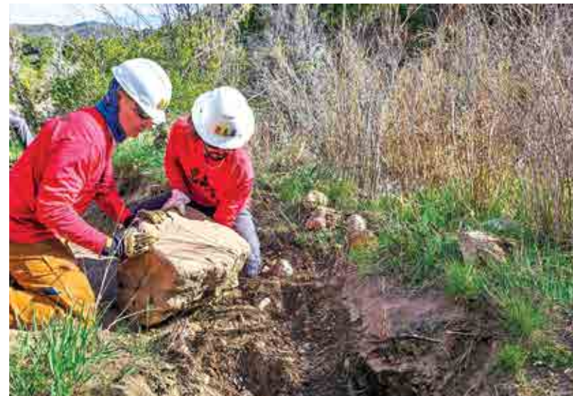
Friends of Nevada Wilderness trail crew leads build rock structures to keep the trail from eroding.
